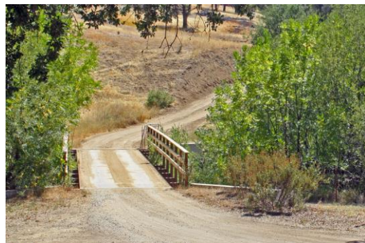
1. Start by the bridge by the Tasting Room.
